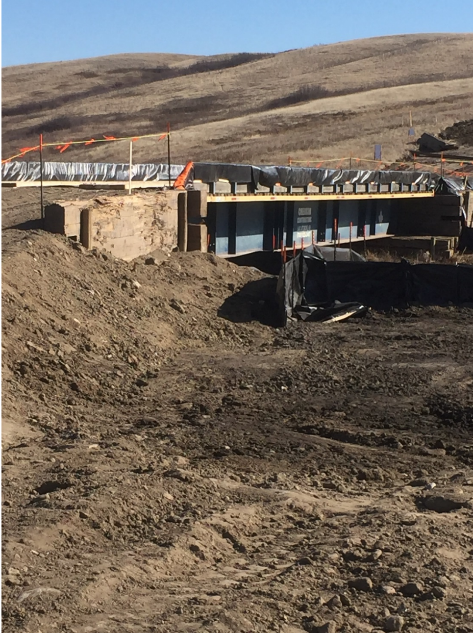
Bridge at Iskwao creek after installation.
