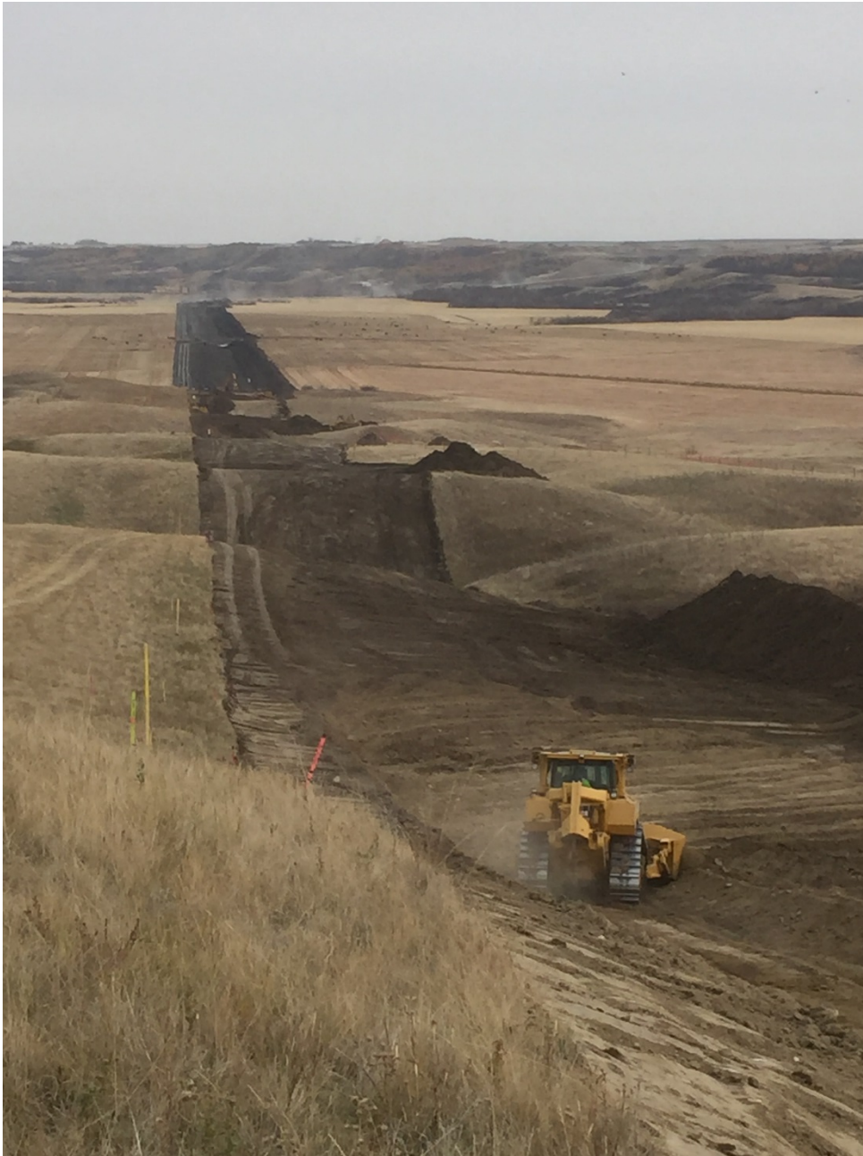
Qu'Appelle valley after it was stripped
