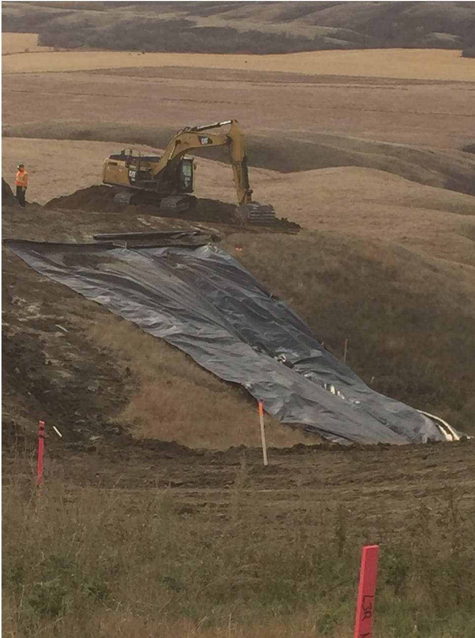
Geo fabric being placed in the valley
